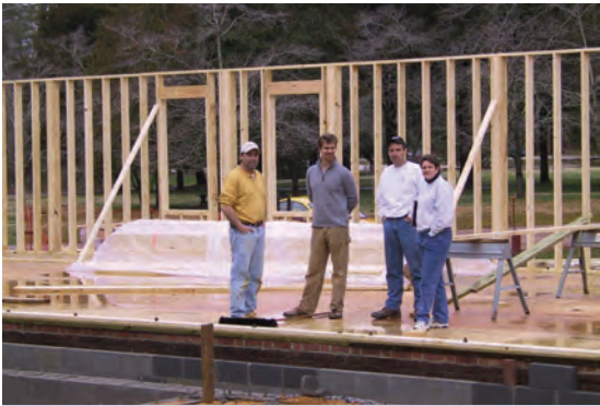
David (second from right), Teresa Bush (far right) and Kenny Ramsey (far left) of Connemara meet with one of the project architects in February 2008 during work on the Chase Center as part of the Foundation's 50th anniversary campaign.
